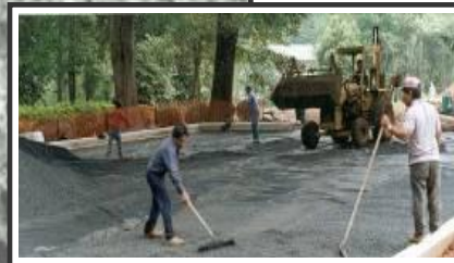
Existing Tree Root Bridging Media Physical Properties Expanded Slate ¾" 100 % Recycled
